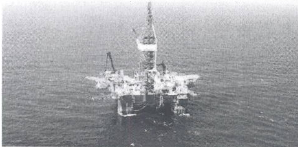
Pemex oil platform in the Gulf of Mexico
